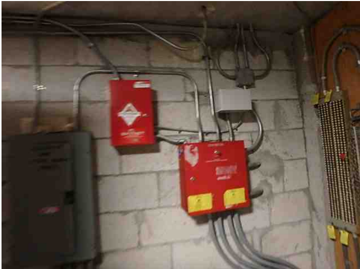
master fire alarm panel
